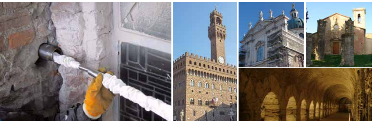
RESTAURATION ET CONSOLIDATION > STRENGTHENING
